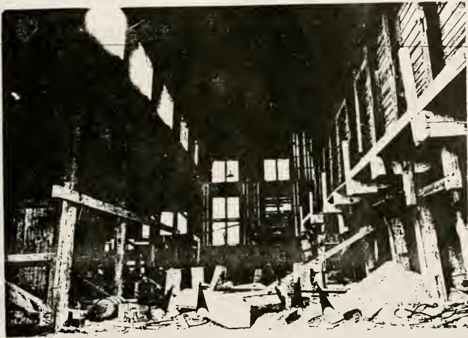
Figure 92. Revenue Mill (structure #34) north view stamp mill and ball mill level - concrete footings for ball mill seen in center (arrows).
